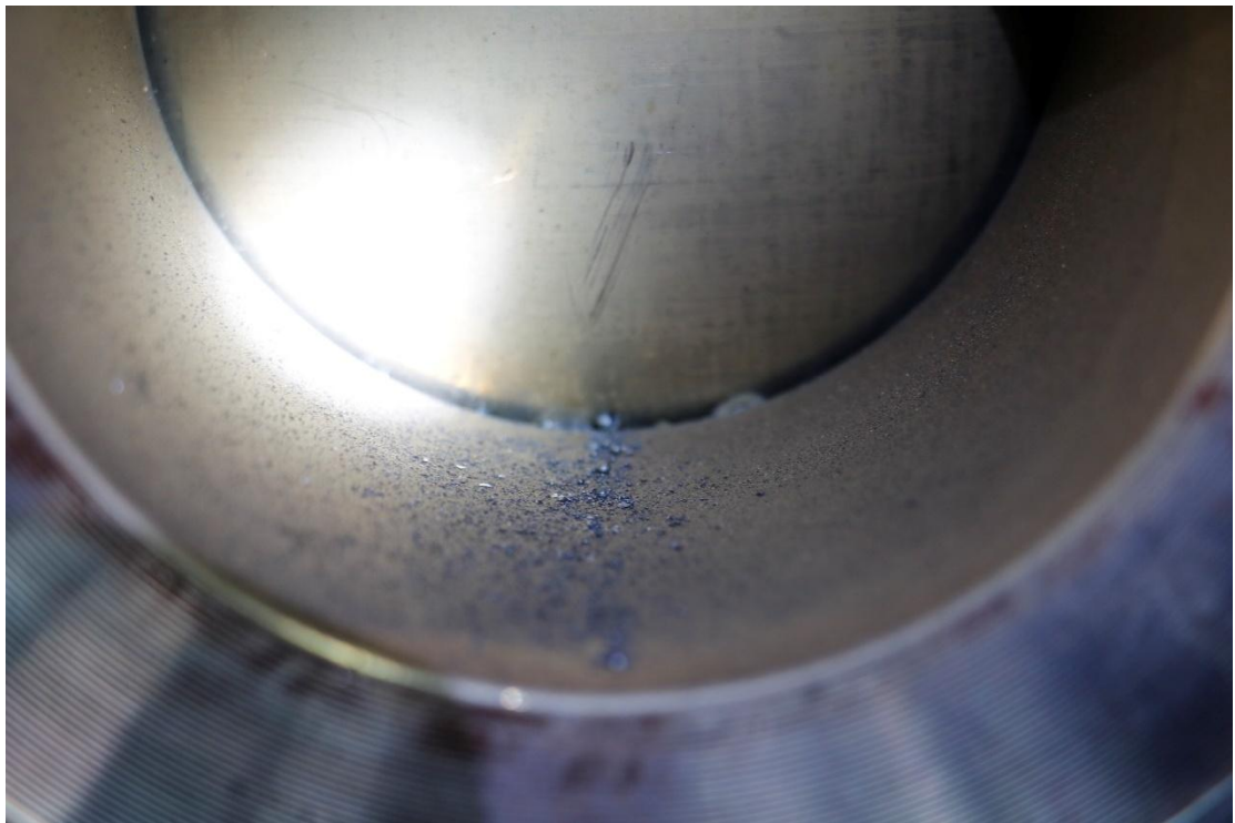
2#压滤机进料管球阀前端焊渣
